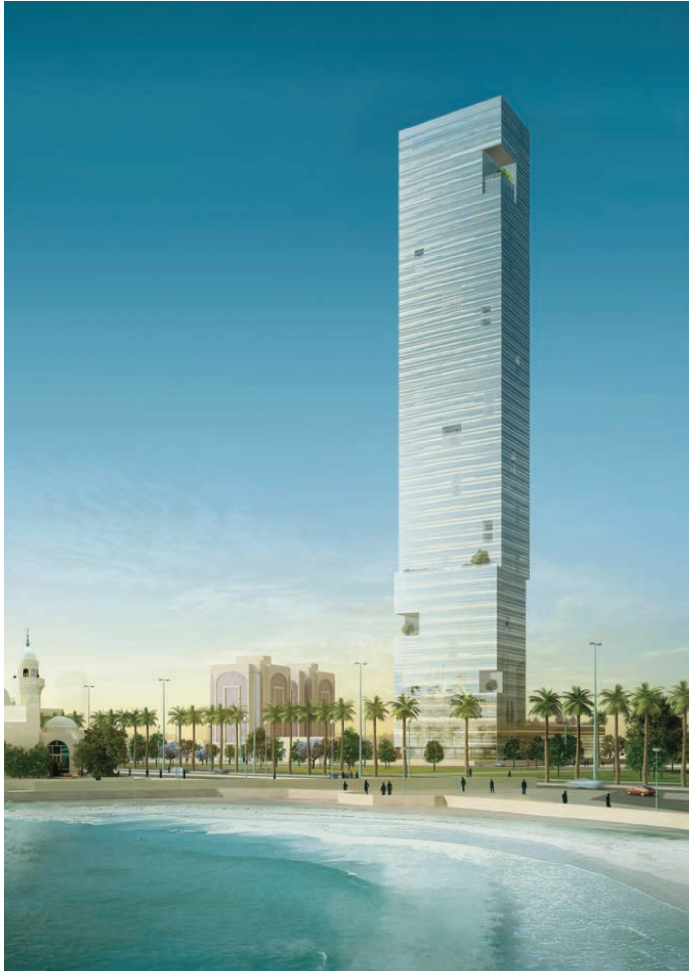
Facing Jeddah's Corniche, the tower benefits from maximum sea exposure
