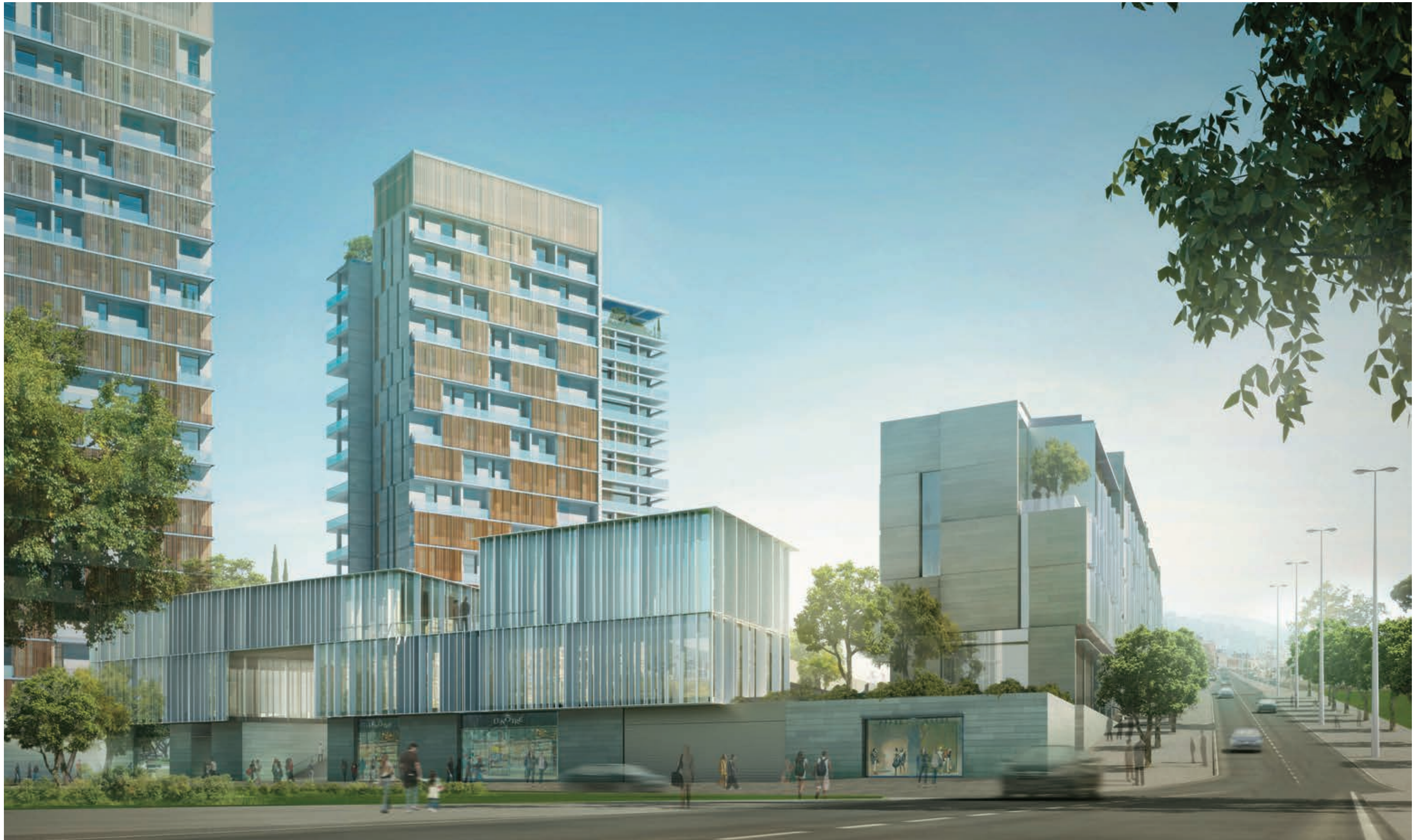
Located along the main street, the office and retail area provides flexible floor space to meet different needs
